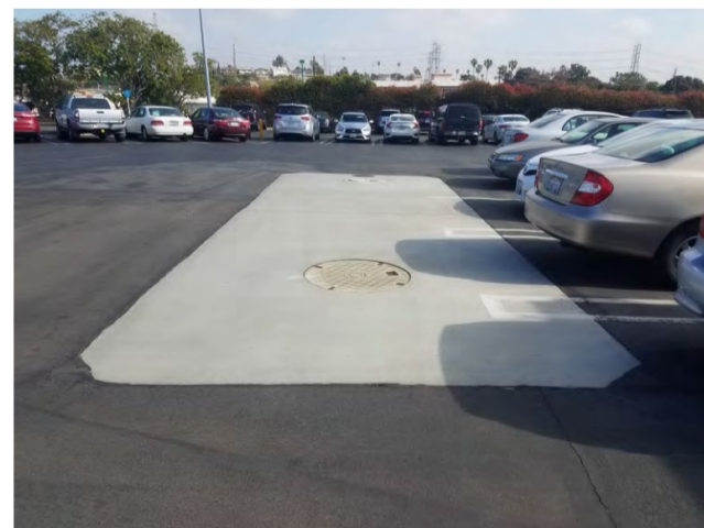
One 10,000-gallon UST is located beneath the existing north surface parking lot on the campus and is associated with back-up generators located within the attached maintenance building.
