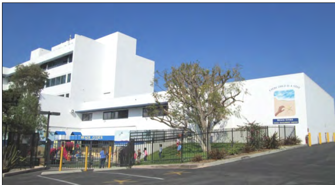
South and east elevations, showing modern addition (behind the tree), view to the northwest.
