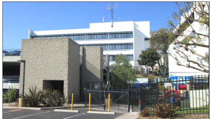
East elevation, view to the west.
