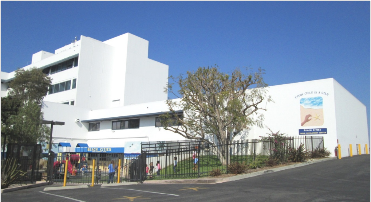
Figure 11: South and east elevations, showing modern addition (behind the tree), view to the northwest (2/6/18).
