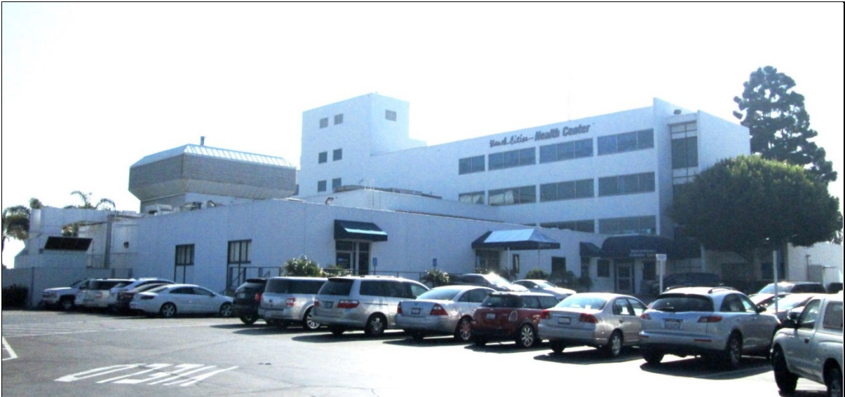
Figure 9: North elevation and addition (circa 1970) to the northwest corner of the building, view to the southeast (2/6/18).
