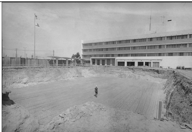
Construction site for new hospital wing, 1968. Source: Gnerre 2015 ( Daily Breeze )
