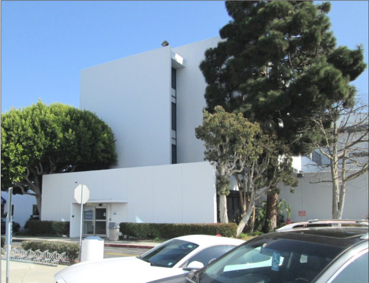
Figure 8: West elevation of the original 1960 building, view to the northeast (2/6/18).
