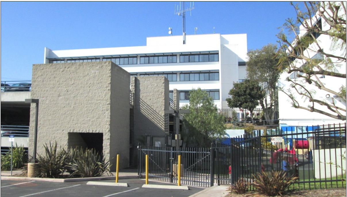
Figure 12: East elevation, view to the west (2/6/18).
