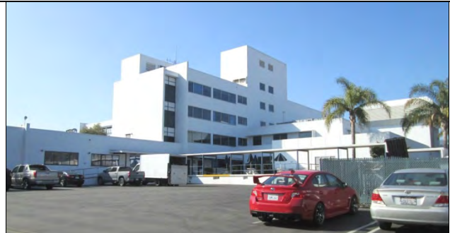
North elevation, view to the southwest. The modern addition is partially shown on the far left of the photograph.
