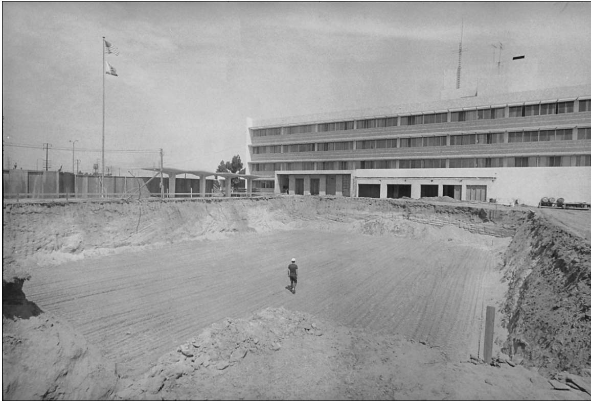
Figure 5: Construction site for new hospital wing, 1968. Source: Gnerre 2015 ( Daily Breeze )
