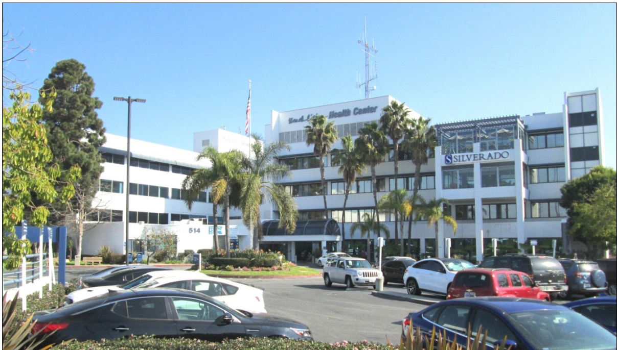
Figure 7: Façade (south and west elevations), view to the northeast (2/6/18).
