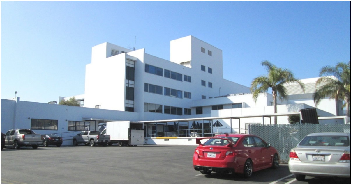
Figure 10: North elevation, view to the southwest (2/6/18). The modern addition is partially shown on the far left of the photograph.
