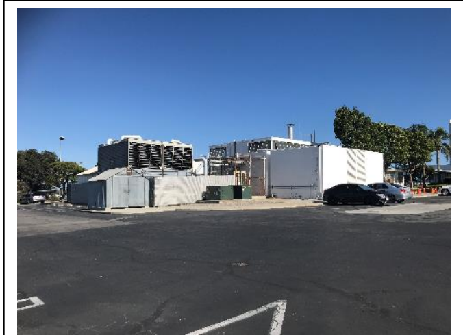
The attached Maintenance Building supports the Beach Cities Health Center and serves as a centralized distribution point for electricity and natural gas utilities.
