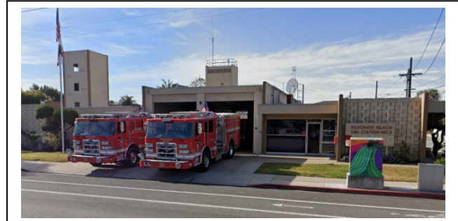
Fire Station No. 2 (pictured above) is located approximately 1.1 miles from the Project site. The RBFD provides fire protection, emergency medical response, and other special services to the population of Redondo Beach.
