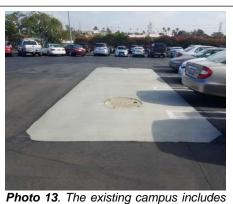
**Photo 13.** The existing campus includes a 10,000-gallon former underground storage tank located beneath the surface parking lot. Soil samples collected in January 2008 during the replacement of piping lines identified the presence of petroleum hydrocarbons that exceeded established maximum concentrations.
